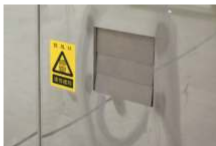
Exhaust hot air outlet
