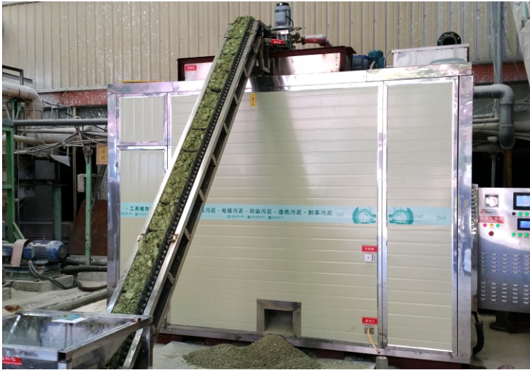
Sludge drying line (6-layers)
